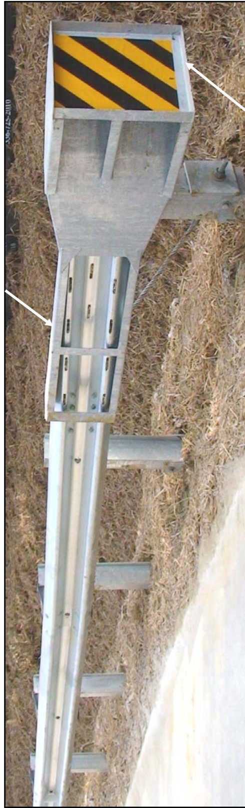
Impact Head Feeder Guide Chute
